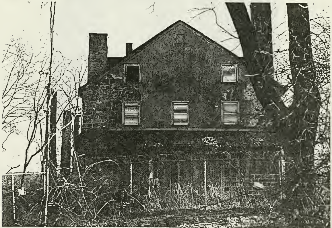
Figure 12: North Elevation of the Pawling/Wetherill House, 1995.
